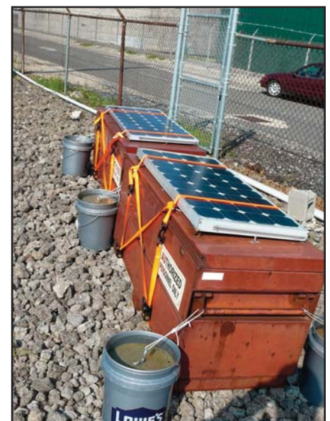
Well boxes moved & stowed on higher ground
