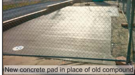
New concrete pad in place of old compound
