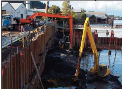
Portland Terminal - excavation & shoring
