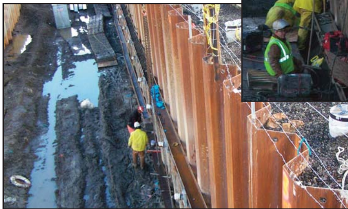
Welders installing tiebacks along the seawall
