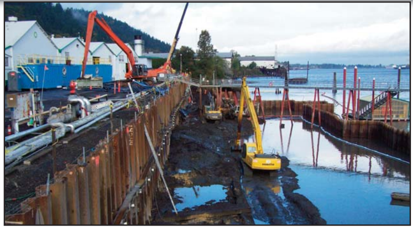
BP's Portland Terminal - seawall & excavators
